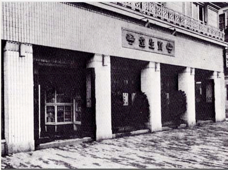
The photo shows the squared, white-tiled pillars of the redesigned Shiseido Parlour building in Ginza, ca. 1920.
