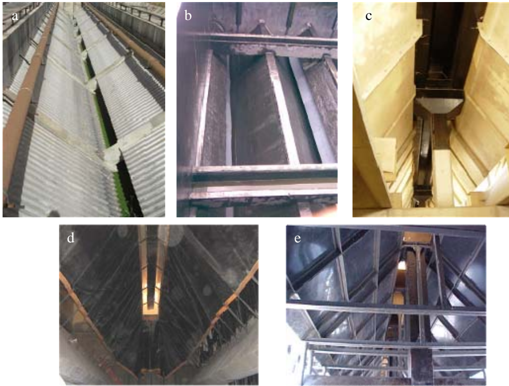
Fig. 4.11. Materials of constructions used for GLS separators: (a) Corrugated iron, (b) concrete, (c) GRP, (d) canvas (PVC-coated woven cotton), and (e) rigid PVC.
